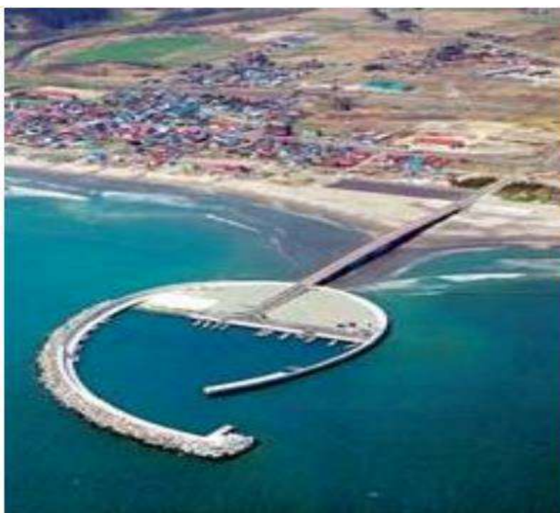
Figure 11: The general view of proposed reclamation and bridge installation (source: Xinhua, 2016)
