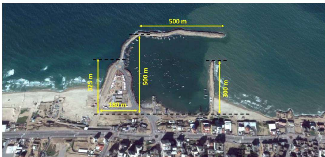
Figure 3: The existing Gaza fishery harbor (source: Google earth, 2016)
