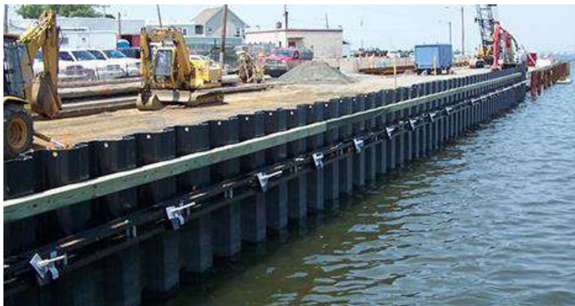
Figure 8: Installation of sheet piles (source: WIKI, 2016)
